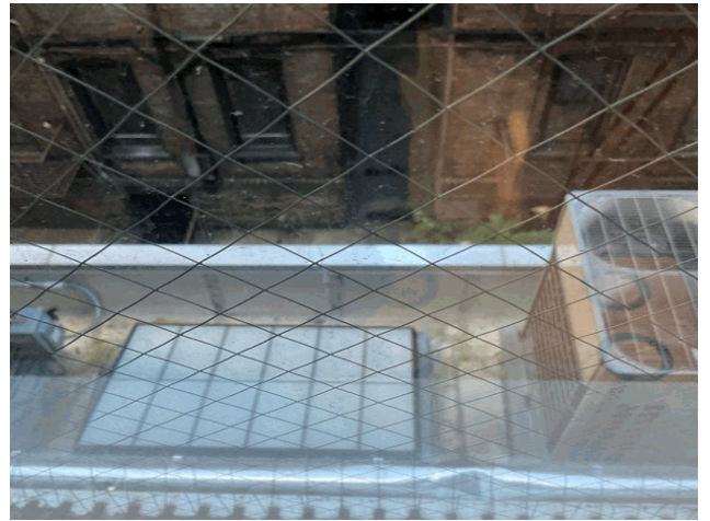
Roof 1 - North View
