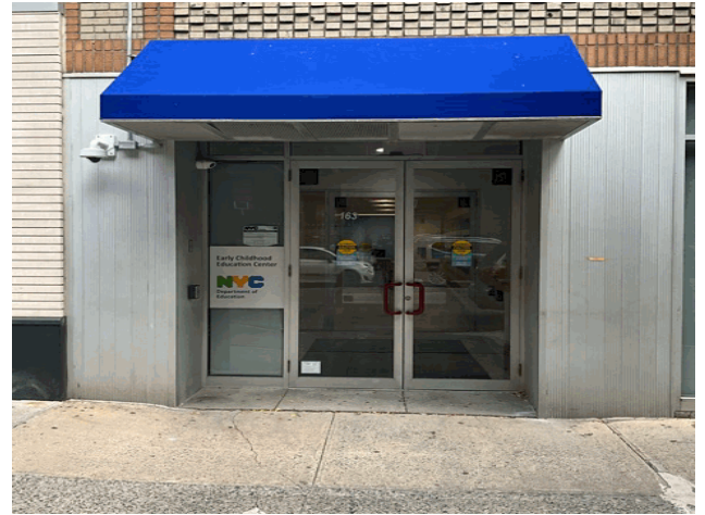
Facade A - East 84th Street
