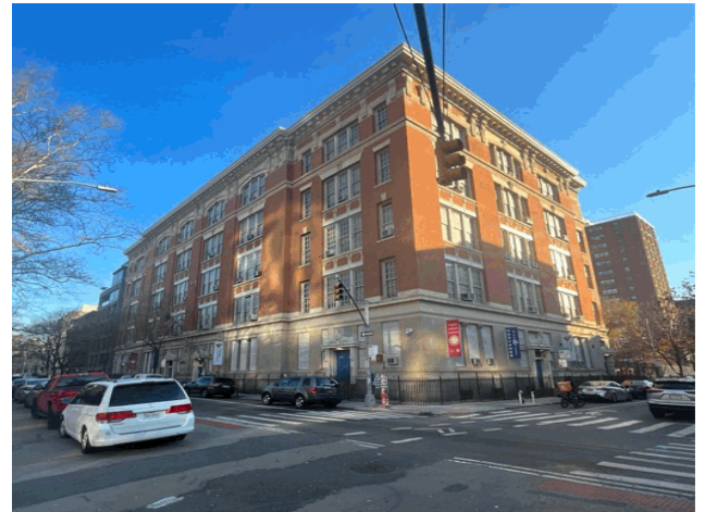
Corner of Stanton Street and Forsyth Street - Northeast View
