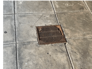
Plaza Deck near Exit 1
