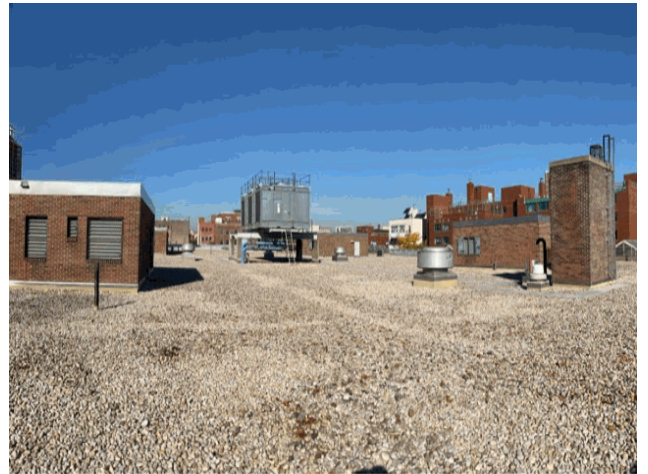
Roof 1 - West View
