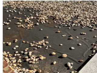
Roof 1 at Bulkhead BH1
