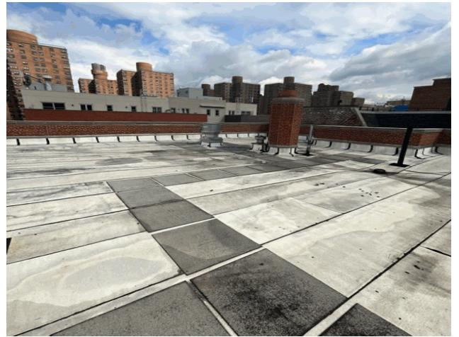
Roof 2 - Northeast View
