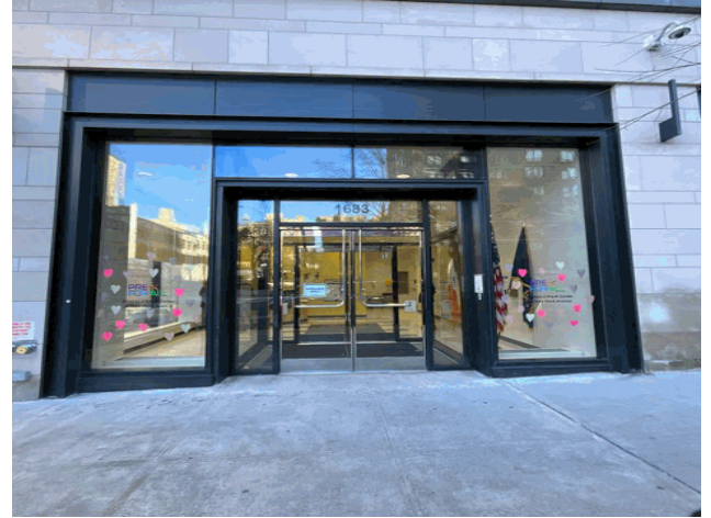
Facade B - 3rd Avenue
