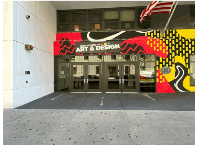
Facade A - East 56th Street
