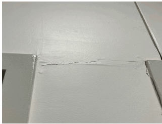
Corridor Near Room 1014
