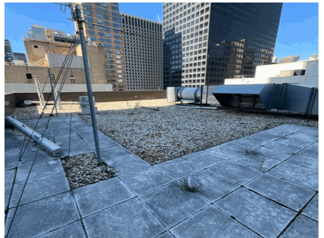
Roof 9 - West View
