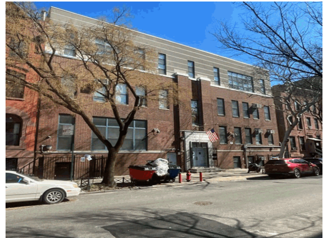
West 132nd Street - East View
