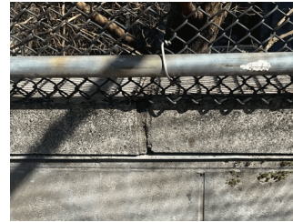
Roof 2 - Facade D
