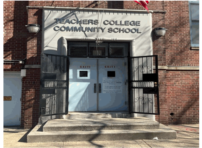
Facade A - West 132nd Street
