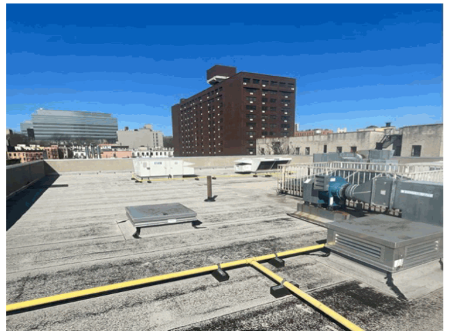
Roof 1 - North View
