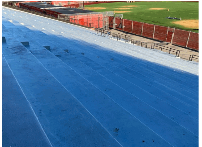
Roof 1 - South View
