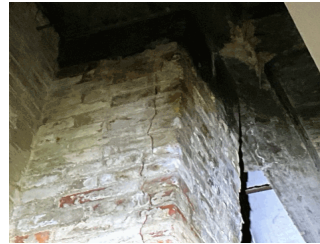
South Pool Mechanical Equipment Room shown, also in Crawl Space at Boiler Room Entrance
