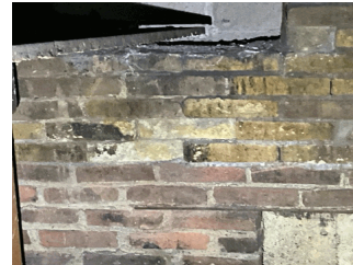
Chimney (at basement)
