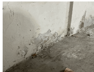
South Pool Mechanical Equipment Room
