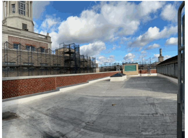
Roof 5 - South View
