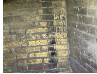
Chimney (At basement)
