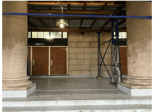
Facade A - Audubon Avenue
