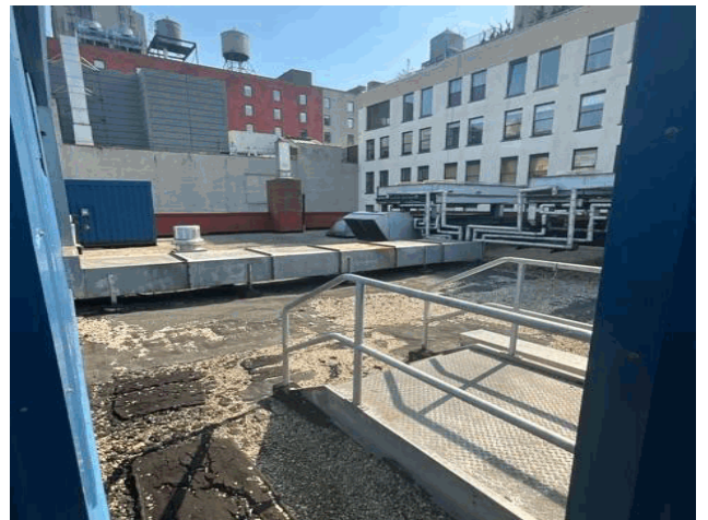
Roof 1 - South View
