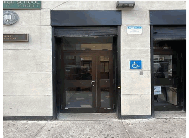
Facade A - West 18th Street
