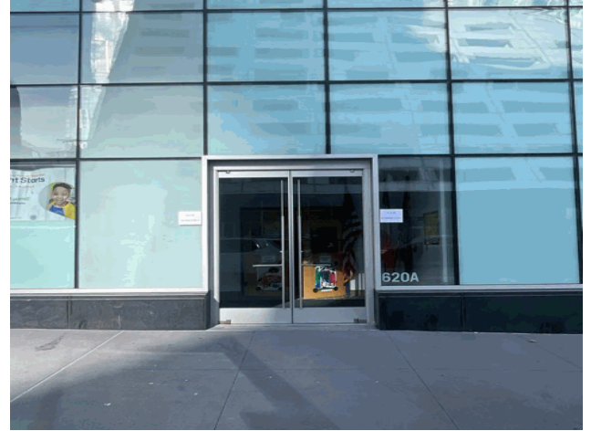
Facade A - West 58th Street
