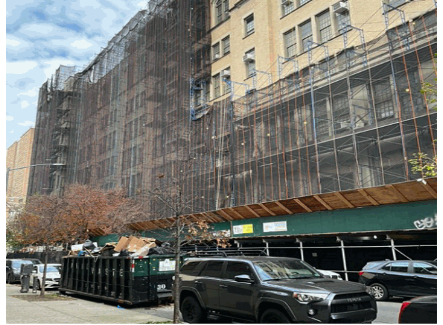
West 18th Street - North View
