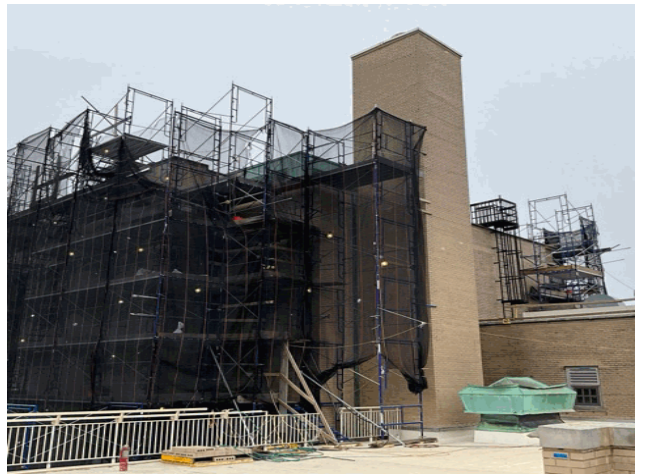
Roof 4 - West View
