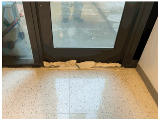
Door to Plaza Deck
