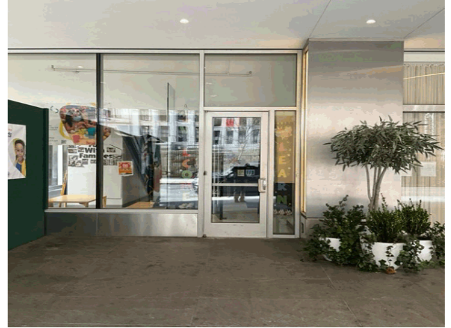
Facade A - Washington Street
