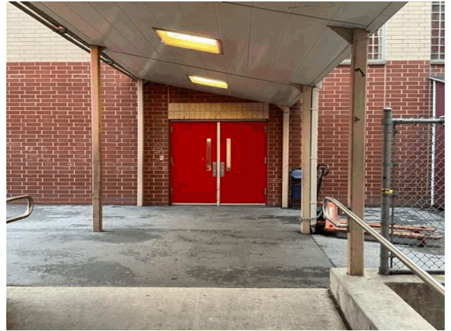
Facade C - Playground
