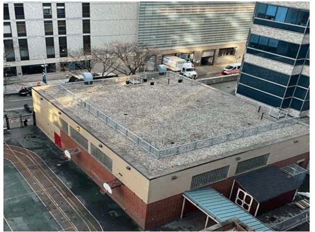
Roof 1 - Northeast View
