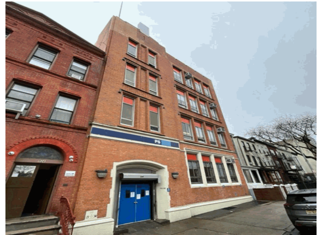
West 153rd Street - South View
