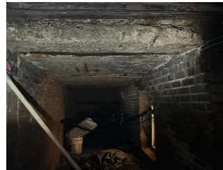
Under Main Entrance Stair (from Areaway AW1)
