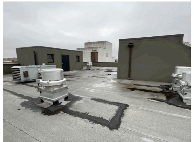
Roof 1 - South View
