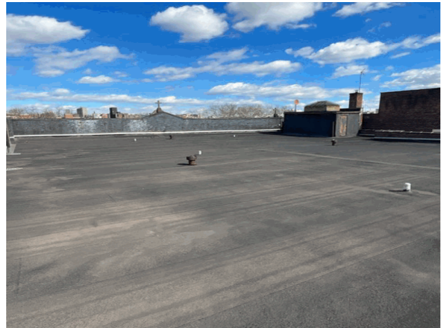
Roof 1 - Northeast View
