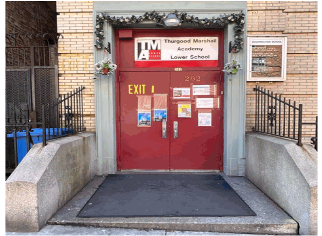
Facade A - West 151st Street
