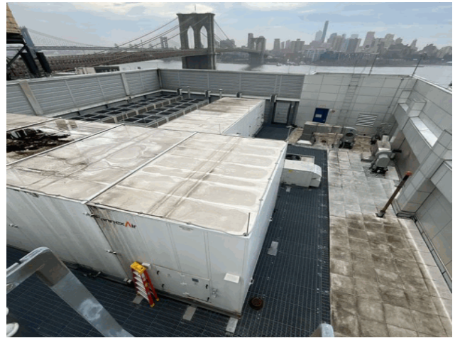
Roof 3 - Southeast View
