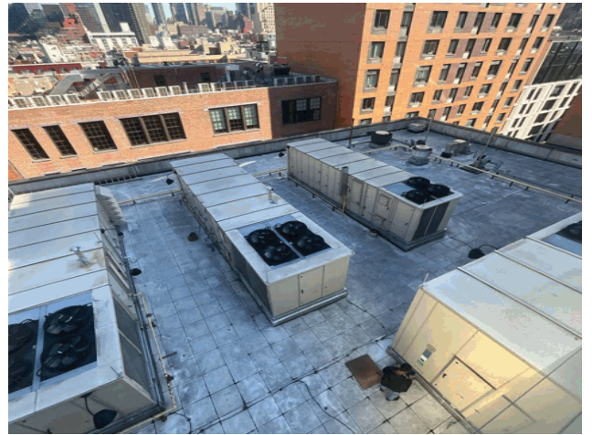
Roof 1 - Northeast View
