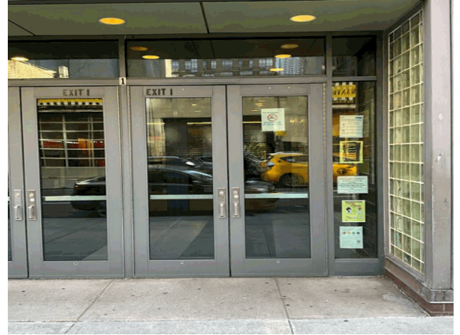
Facade A - West 44th Street
