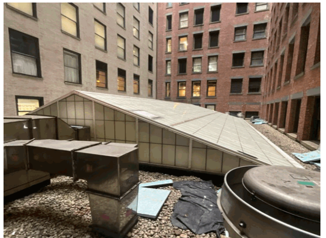
Roof 1 - West View
