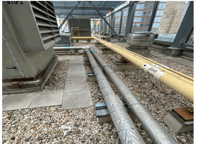
Roof 2 - North View
