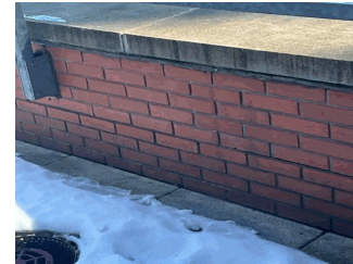
Roof 4 - Facade B
