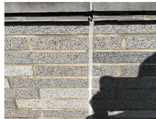
Roof 1 at Facade C
