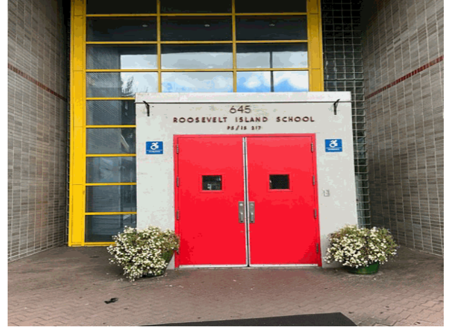
Facade A - Main Street
