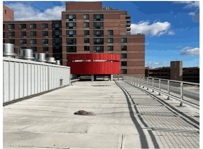
Roof 1 - North View
