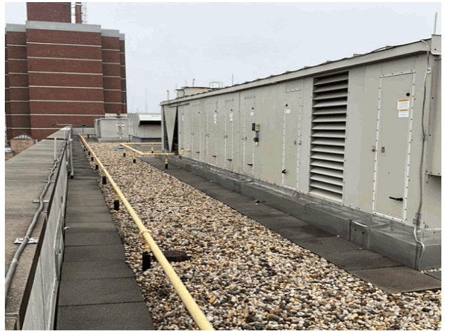
Roof 1 - East View
