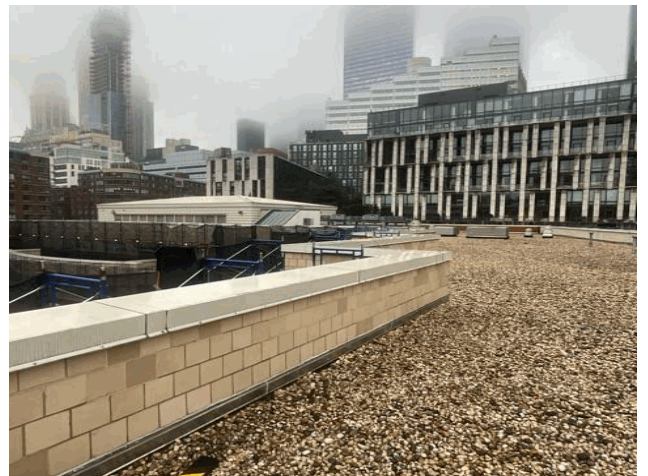
Roof 1 - Southeast View
