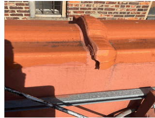
Roof 1 - Facade C
