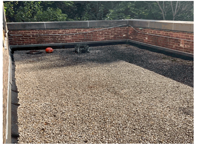
Roof 5 - East View
