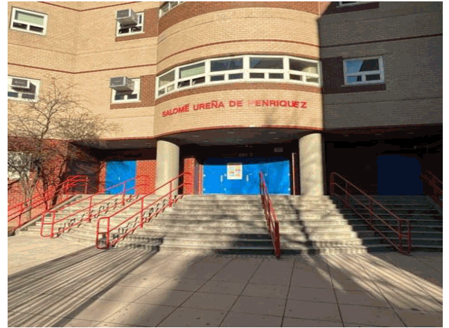
Facade A - West 196th Street
