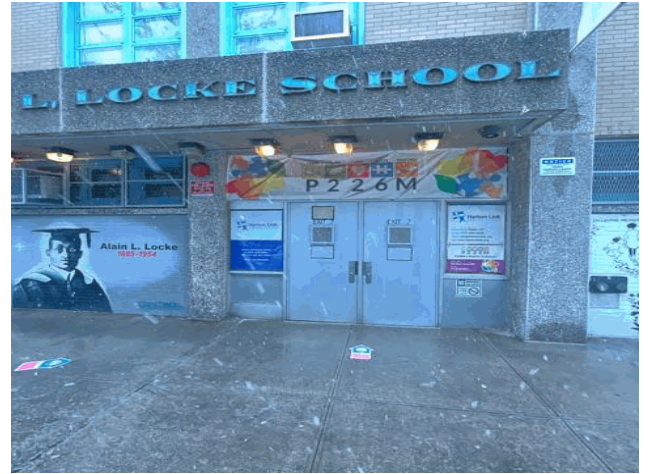
Facade A - West 111th Street
