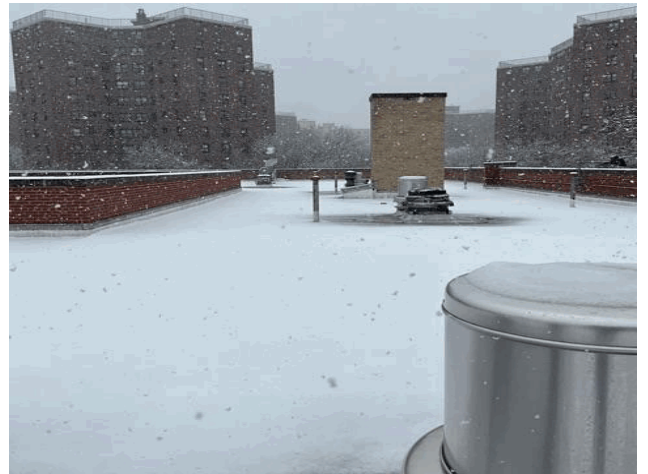
Roof 1 - Northeast View
