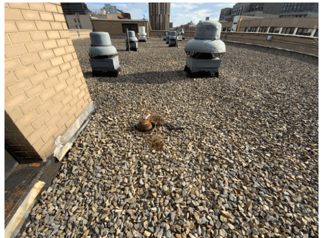
Roof 5 - East View
