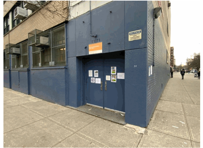
Facade E - West 118th Street
