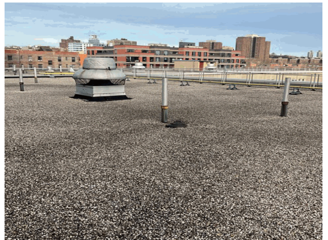
Roof 1 - North View
