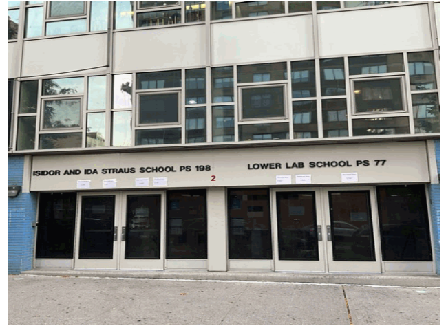
Facade A - 3rd Avenue
