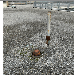
Roof 1 - West View
