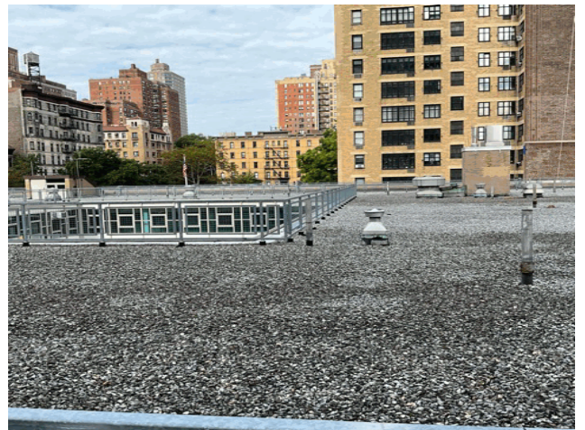
Roof 1 - West View
