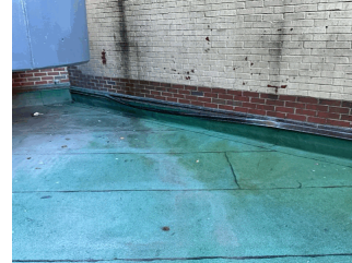
Roof 1 at Facade A
