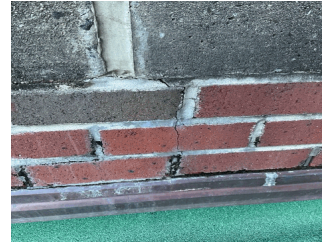
Roof 1 at Facade E
