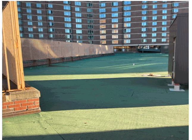
Roof 1 - North View
