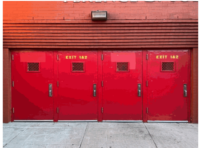
Facade A - West 133 Street
