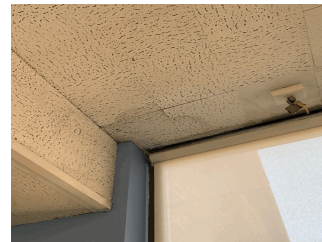
Corridor Near Stair A/3 shown, also in Corridor Near Room 382
