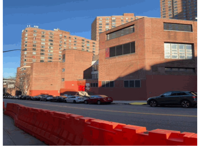
West 133 Street - North View
