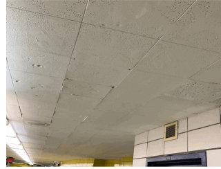
Corridor near Room 354
