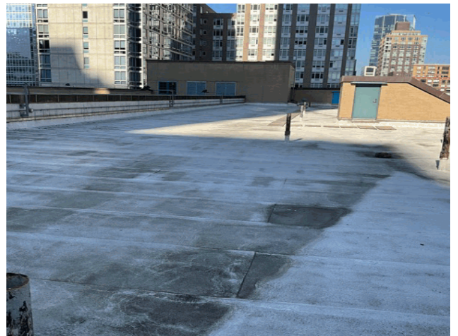
Roof 1 - East View
