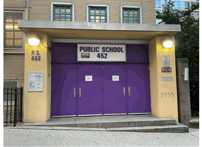
Facade A - West 61st Street
