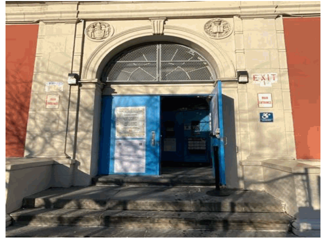
Facade A - East Houston Street (Play Yard)
