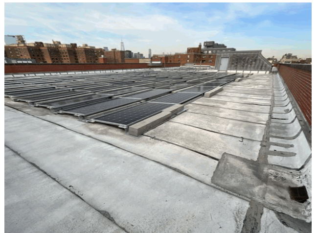
Roof 1 - West View
