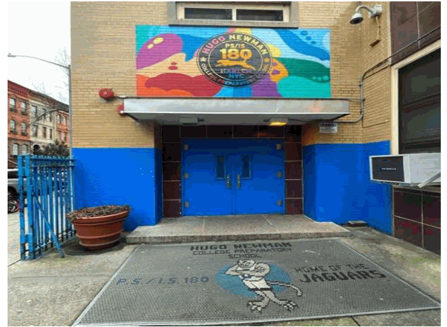
Facade A - West 120th Street
