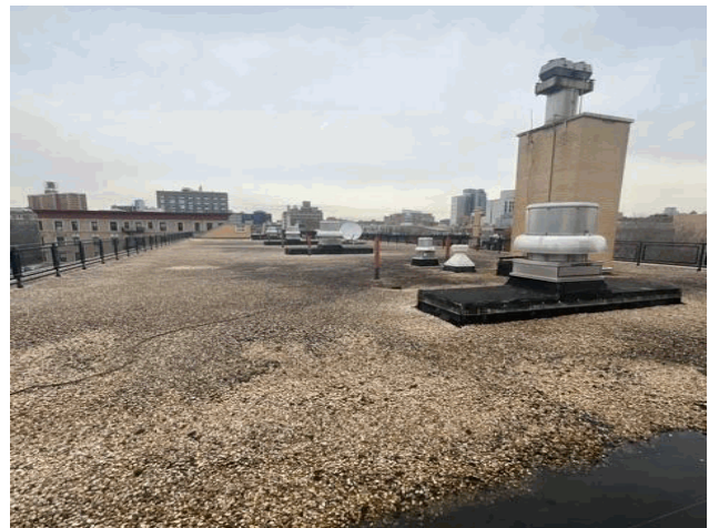
Roof 2 - Northeast View
