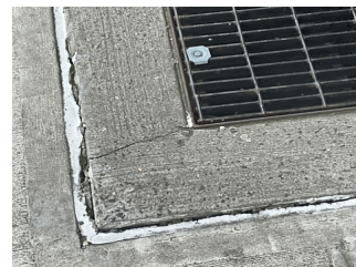
Areaway AW2 No photo recorded
