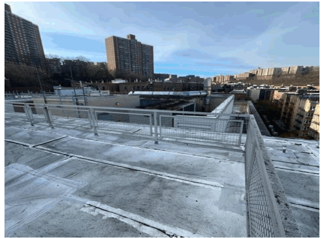
Roof 2 - Southeast View
