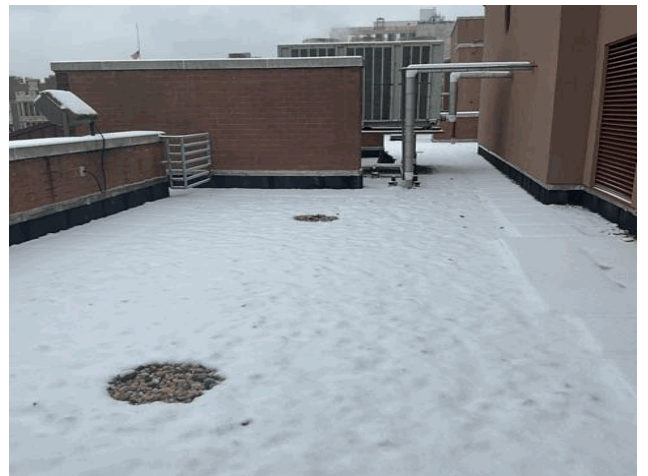
Roof 1 - Northeast View
