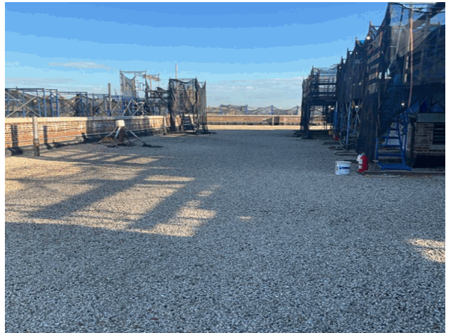
Roof 1 - Northeast View
