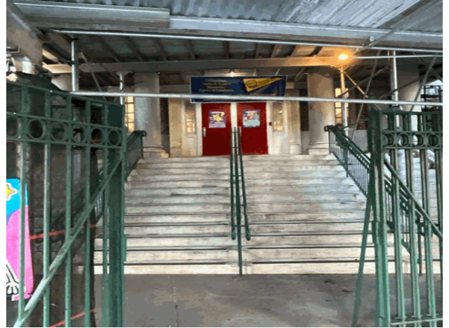
Facade A - Fort Washington Avenue
