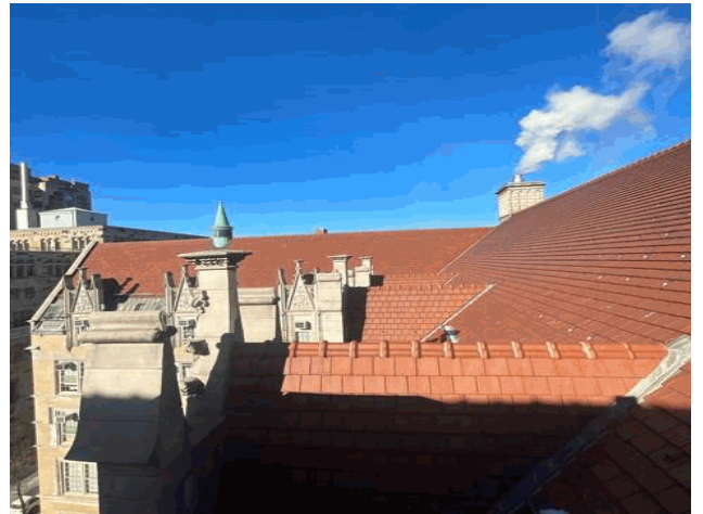
Roof 2 - West View
