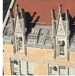
Roof 1 at Skylights
