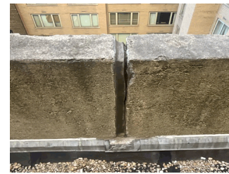
Roof 11 - Facade B
