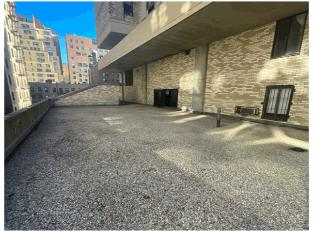
Roof 1 - Northeast View
