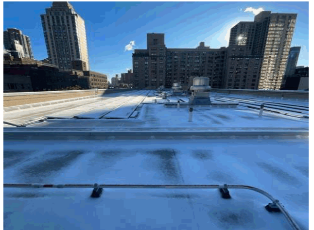
Roof 1 - East View
