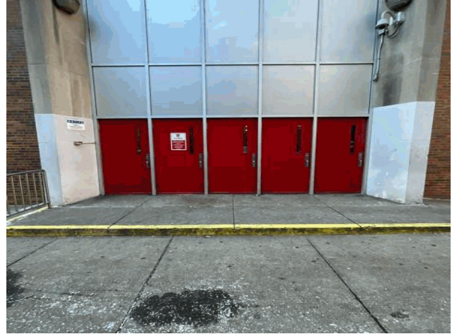
Facade A - East 76th Street
