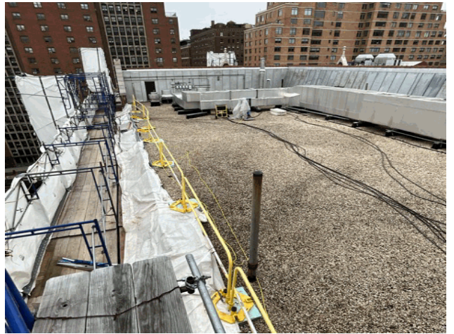
Roof 1 - Northwest View
