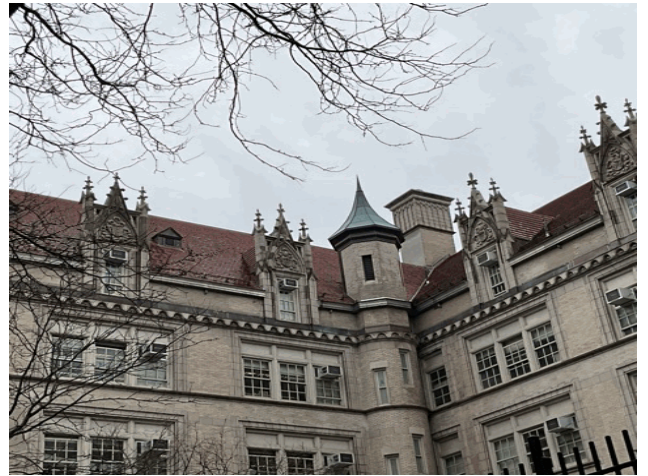
Roof 1 - South View
