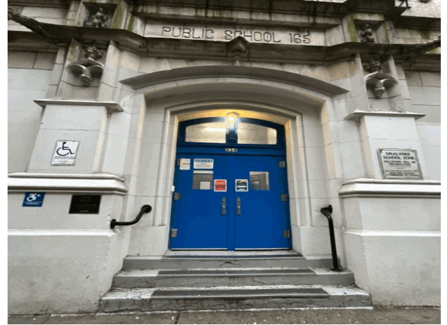
Facade A - West 109th Street
