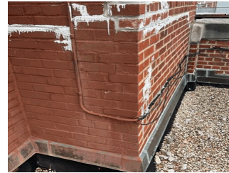
Roof 1 - Facade H
