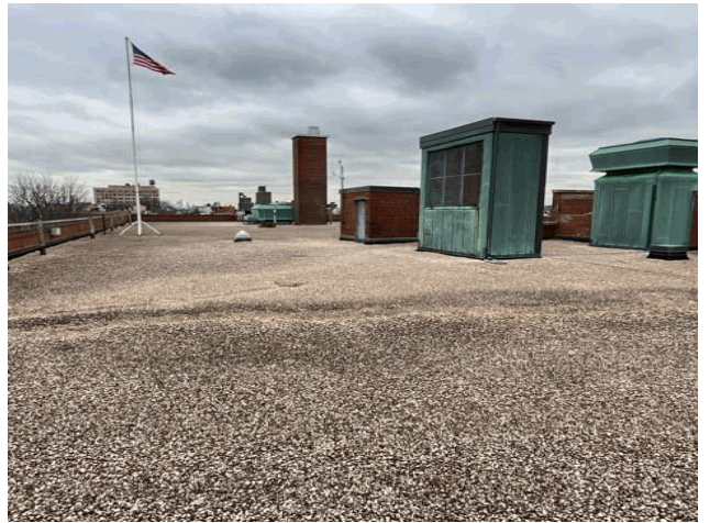
Roof 1 - Southwest View
