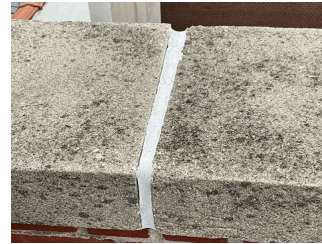
Roof 1 - Facade D
