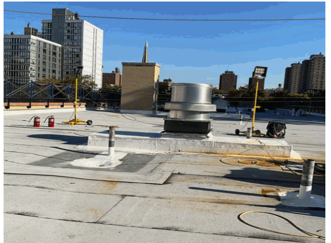
Roof 1 - North View
