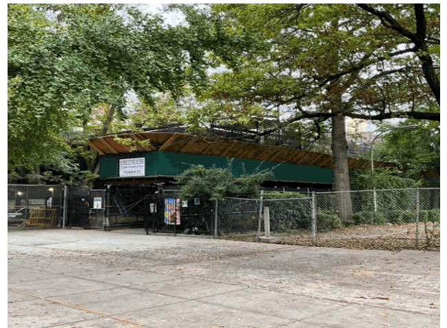
West 97th Street - South View
