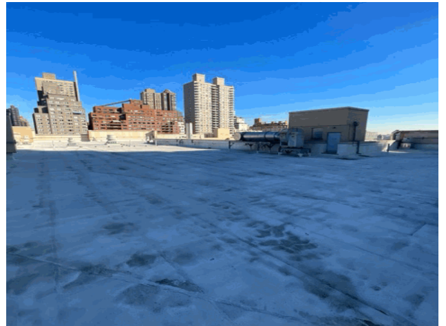
Roof 1 - Northeast View
