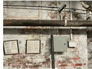
Chimney at Basement
