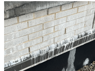
Roof 1 - Facade F
