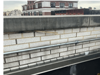
Roof 1 - Facade J
