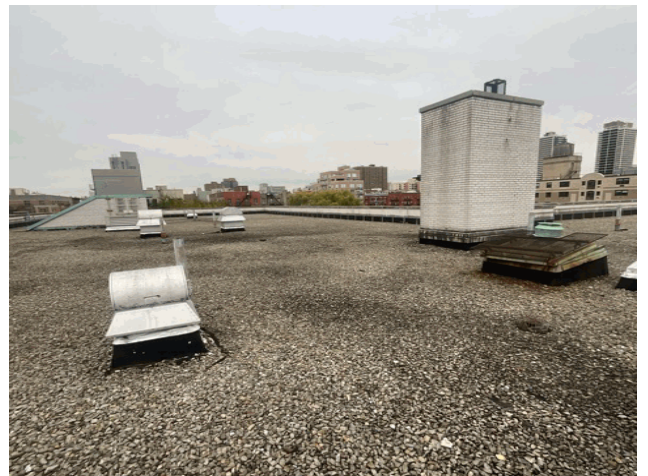
Roof 1 - Northwest View
