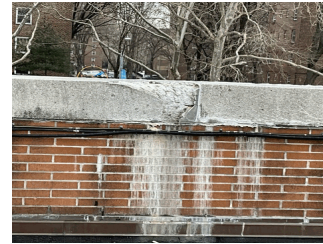
Roof 1 - Facade A
