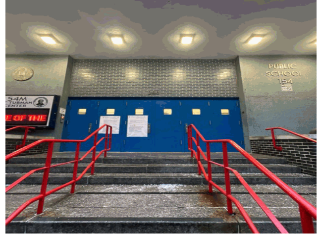
Facade A - West 127th Street
