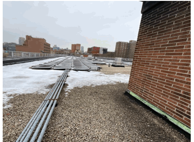
Roof 4 - Northwest View
