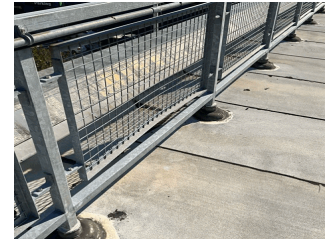
Roof 1 at Facade H
