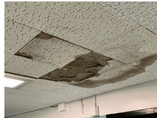
Corridor near Room 401 shown, also in Room 403
