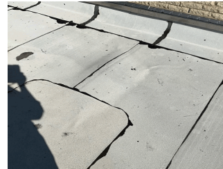
Roof 1 near Bulkhead BH1
