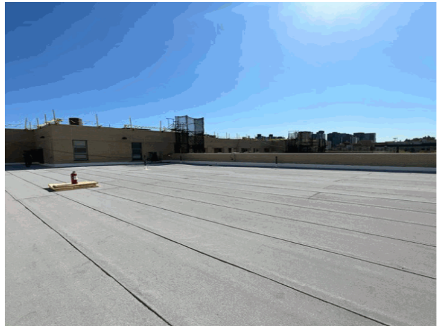
Roof 9 - East View
