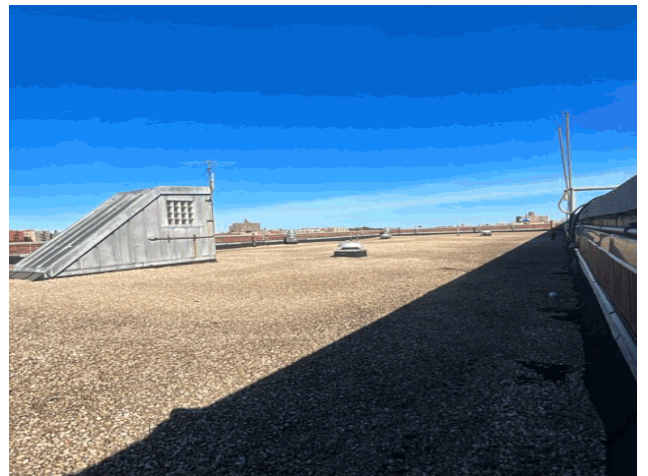
Roof 5 - Northeast View
