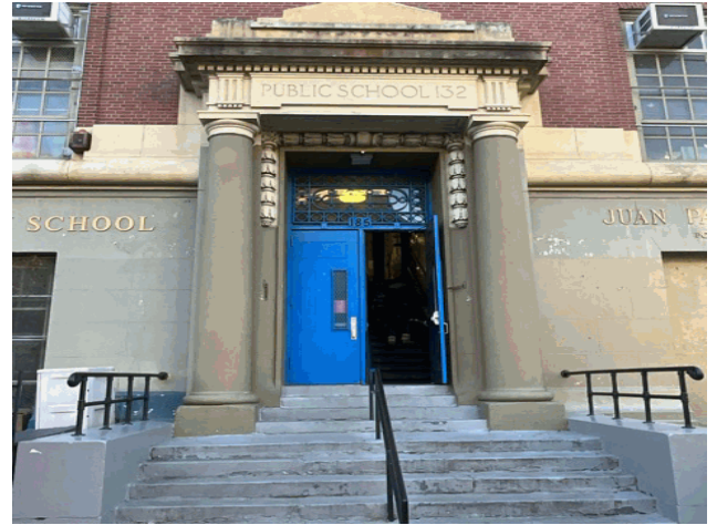
Facade A - Wordsworth Avenue
